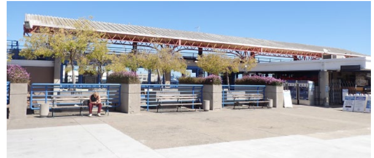
Current Port fencing condition: Terminal Southwest
