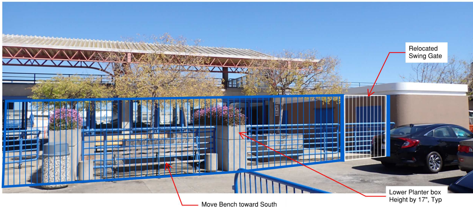
SFFT (Southeast side) (Post Fencing Improvement and Swing Gate Relocation)
