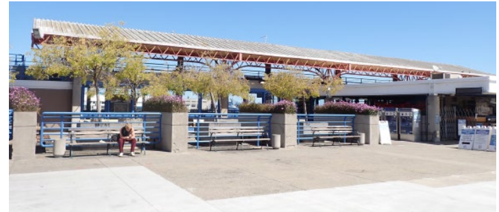
Current Port fencing condition: Terminal Southwest
