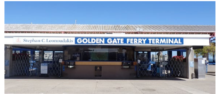
Current Port fencing condition: South building
