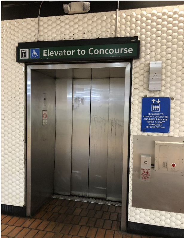
Figure 7. Door vandalism and deterioration of platform elevator at Powell St. station, December 2021.
