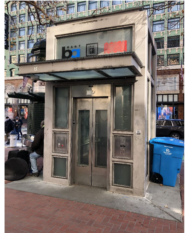
Street elevator at Powell St station, December 2021.
