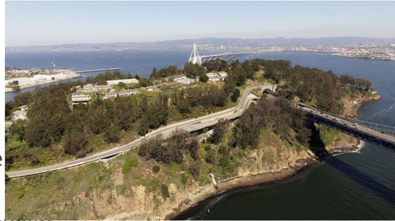
West Side Bridges.
