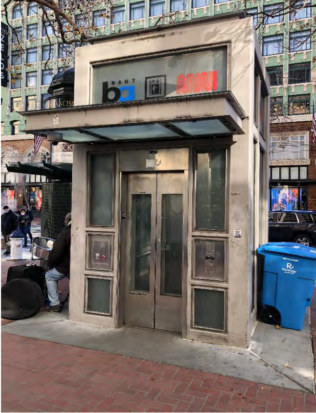
Figure 3. Street elevator at Powell St. station, December 2021.
