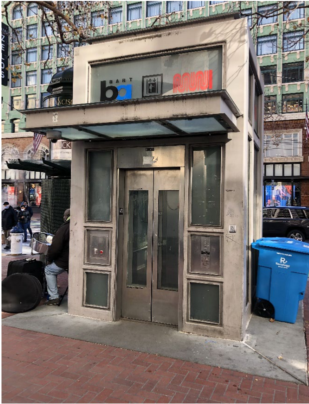
Figure 3. Street elevator at Powell St. station, December 2021.
