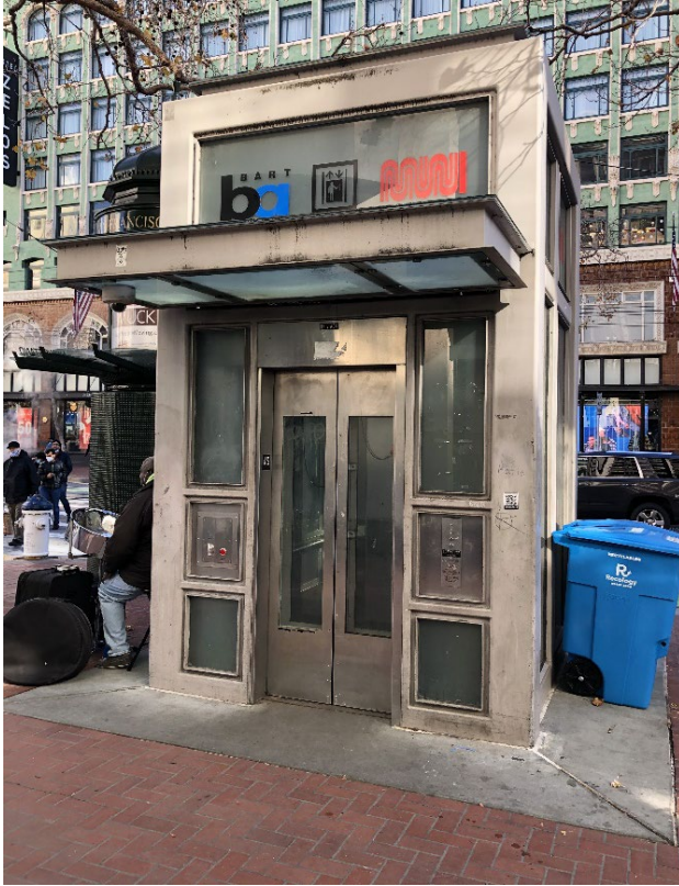
Figure 3. Street elevator at Powell St. station, December 2021.
