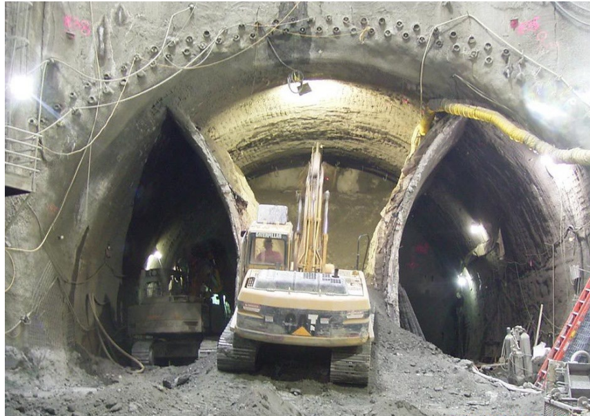
Figure 7-2. SEM Construction Example, Showing Pipe Support Over Tunnel Crown and Sequentially Excavated Tunnel Drifts (Beacon Hill Station, Sound Transit, Seattle)
