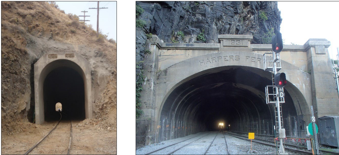
Figure 7-6. Examples of Single and Multitrack Portals
