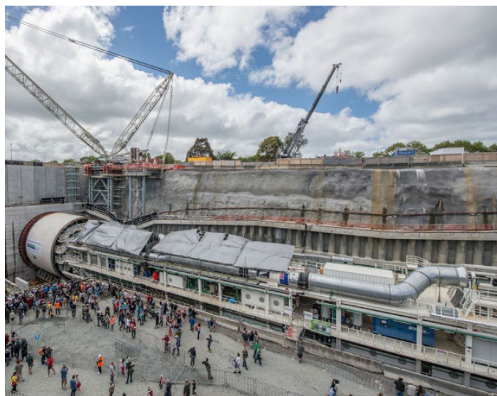
Figure 7-7. Example of a TBM Set Up and Ready to Excavate into a Headwall (46-foot-diameter TBM, Waterview, NZ)
