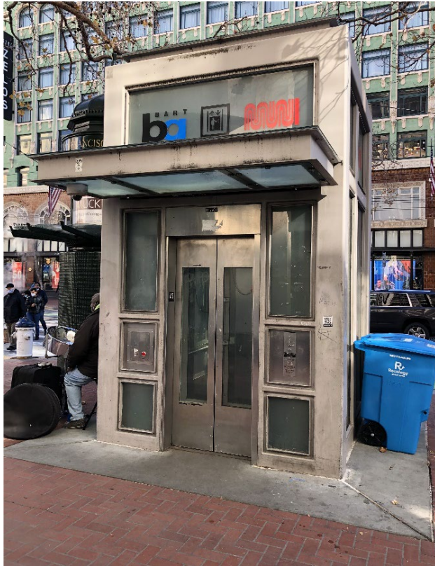
Figure 5. Street elevator at Powell St. Station, December 2021.
