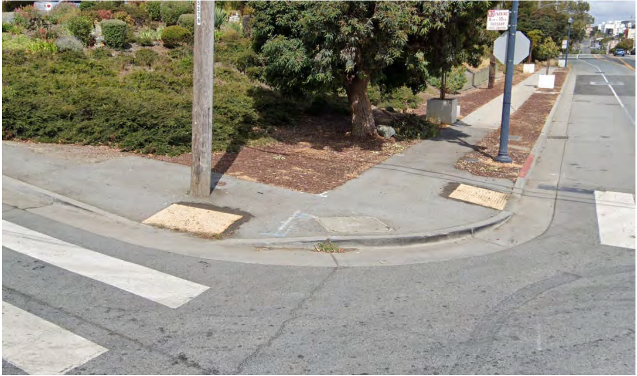
PHOTO 7 – INNES AND DONAHUE – WEST RETURN (Google Streetview image from June 2021)
