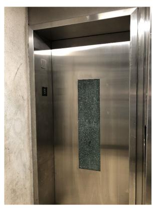
Figure 10. Shattered window glass of platform elevator at Civic Center Station, December 2021.
