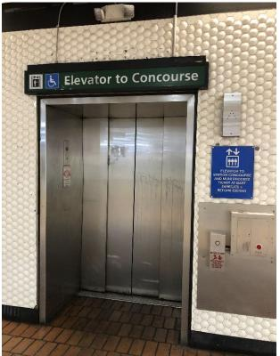
Figure 9. Door vandalism and deterioration of platform elevator at Powell St. Station, December 2021.
