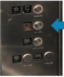
Figure 8. Vandalism to destination buttons at Civic Center Station street elevator, December 2021.
