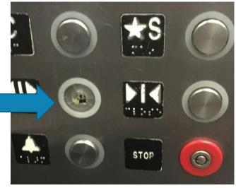
Figure 7. Vandalism to destination buttons at Powell St. Station platform elevator, December 2021.
