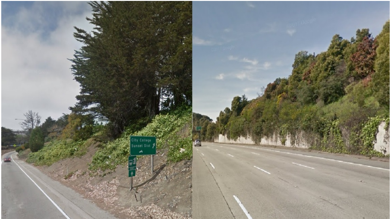
Sloped area of the existing off ramp (shown on left) that would be replaced by an extra travel lane and retaining wall. A typical retaining wall along the I280 corridor is shown at right.
