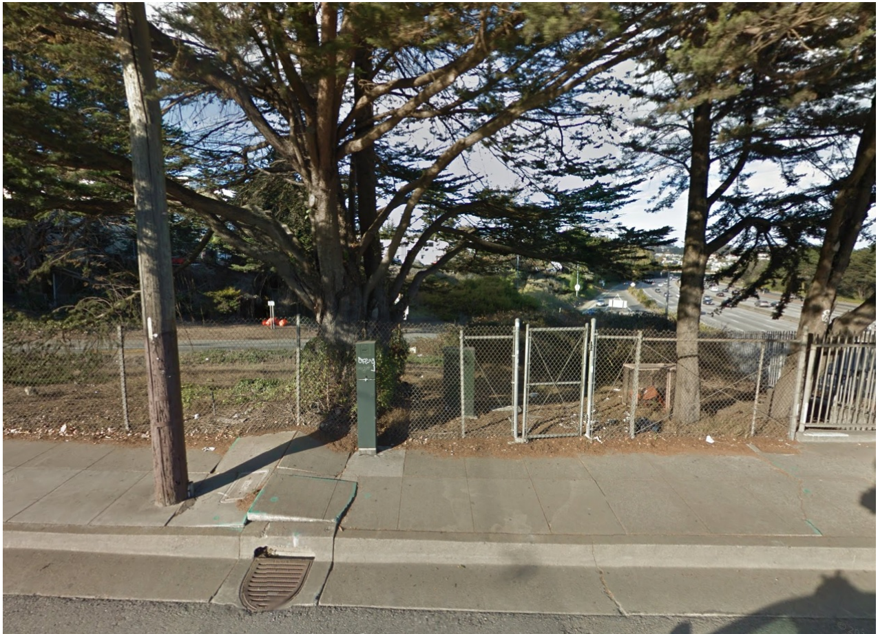
The cypress trees that will be removed by the proposed intersection improvements. Note the heaving of the sidewalk that is occurring.
