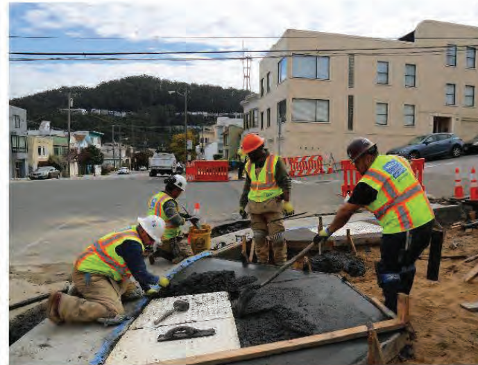
Curb ramp with no sub-sidewalk basement below
