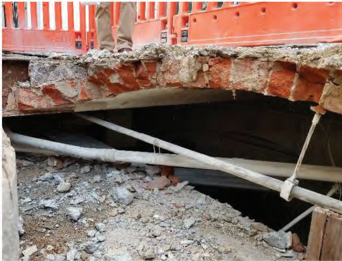
Curb ramp with a sub-sidewalk basement below
