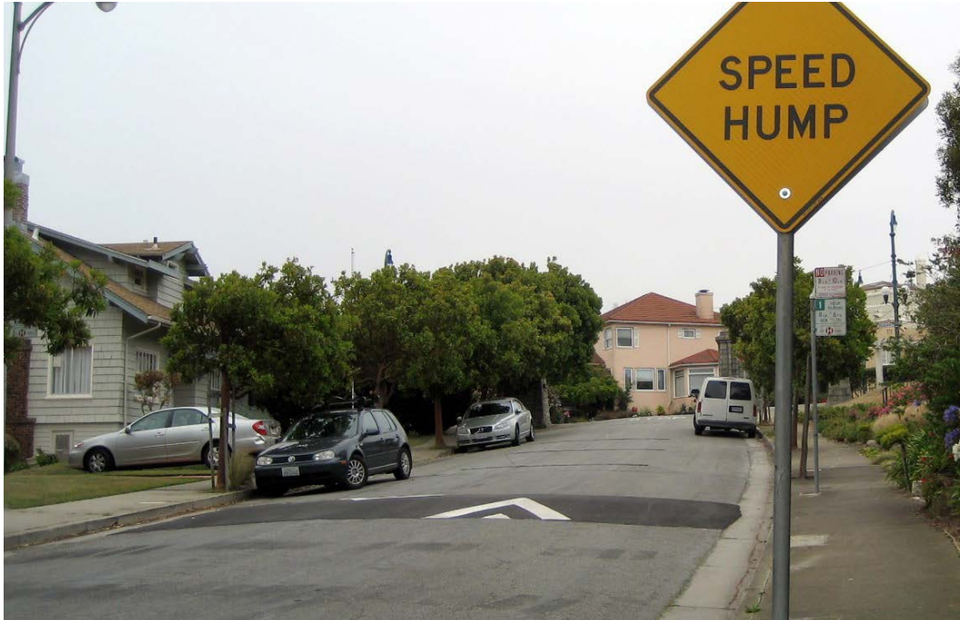
Figure 3-1. Speed humps reduce vehicle speeds
