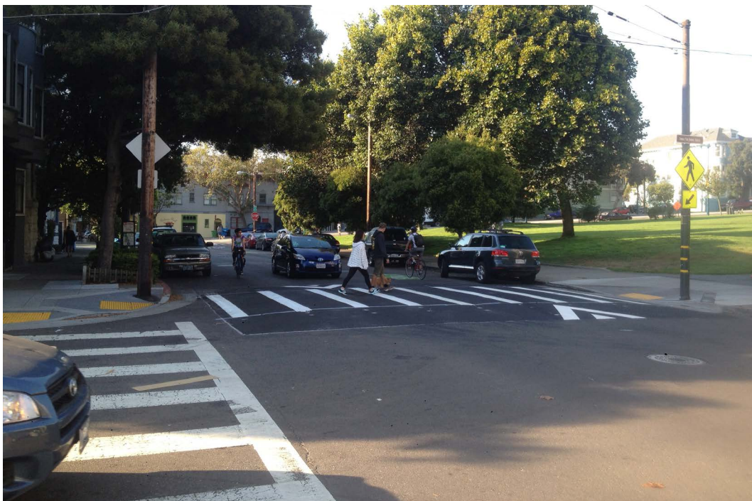
Figure 3-2. Raised crosswalks slow vehicles in areas of significant pedestrian presence
