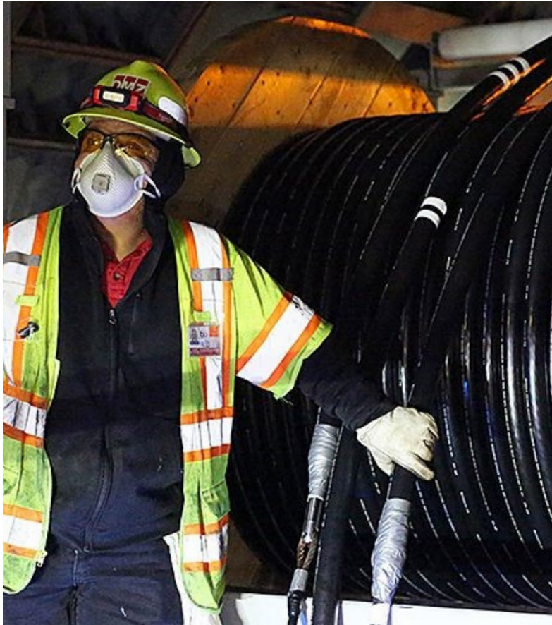
34.5kv Cable Replacement/Upgrade & Traction Power Substations
