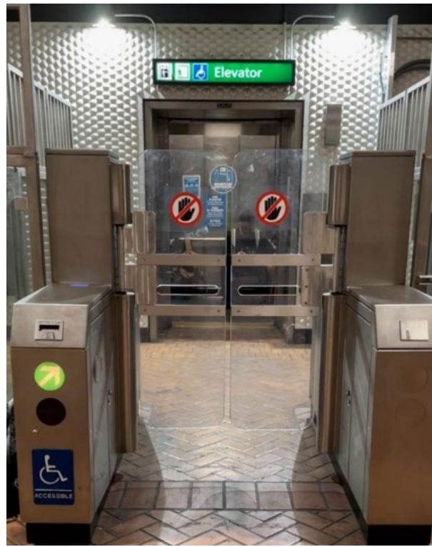
Montgomery St. Station Accessible Fare Gate
