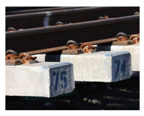
Cement ties like those to the right are replacing aging wooden ties and help to provide a more stable ride.
