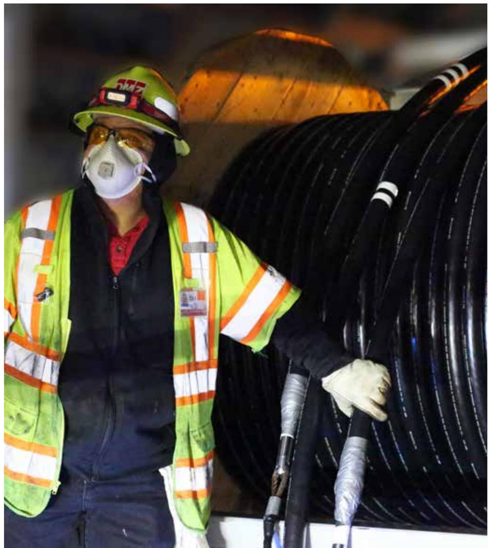
34.5 kV electrical cable used to power trains about to be installed in downtown San Francisco.
