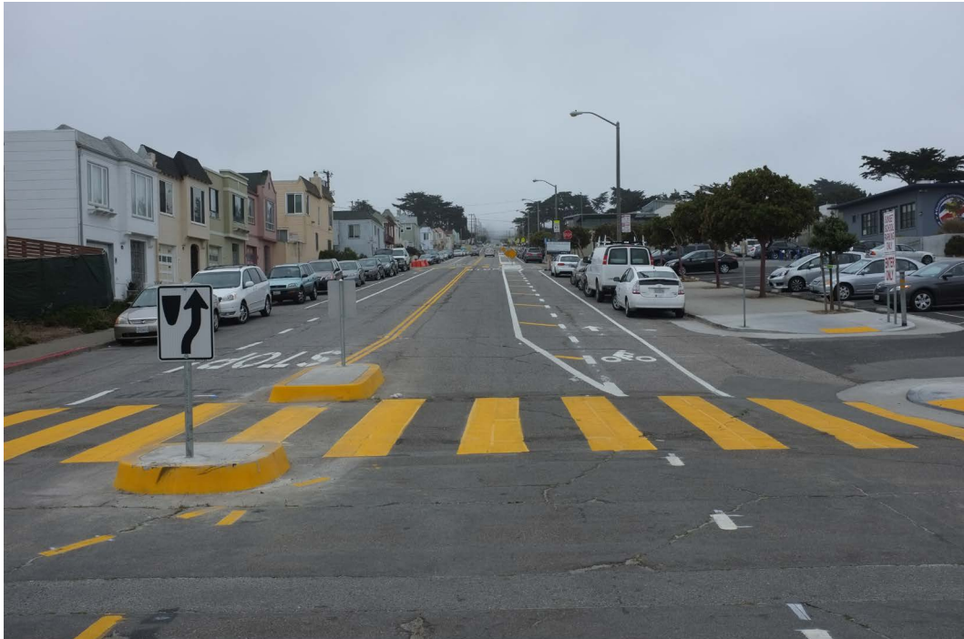
Figure 3-3. Bike lanes designate a portion of the roadway for bicycle use.
