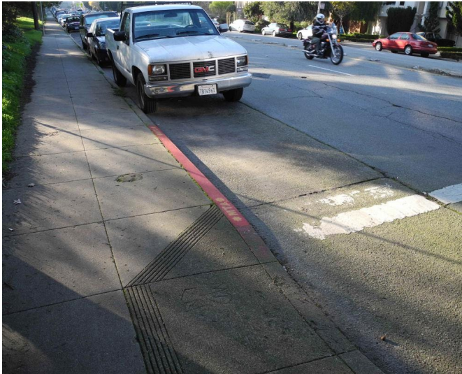
Figure W. Painted safety zones slow down vehicles that are turning at the intersection and improve visibility between drivers and pedestrians.
