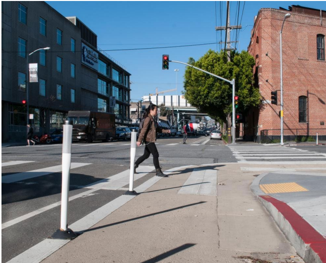
Figure W. Painted safety zones slow down vehicles that are turning at the intersection and improve visibility between drivers and pedestrians.
