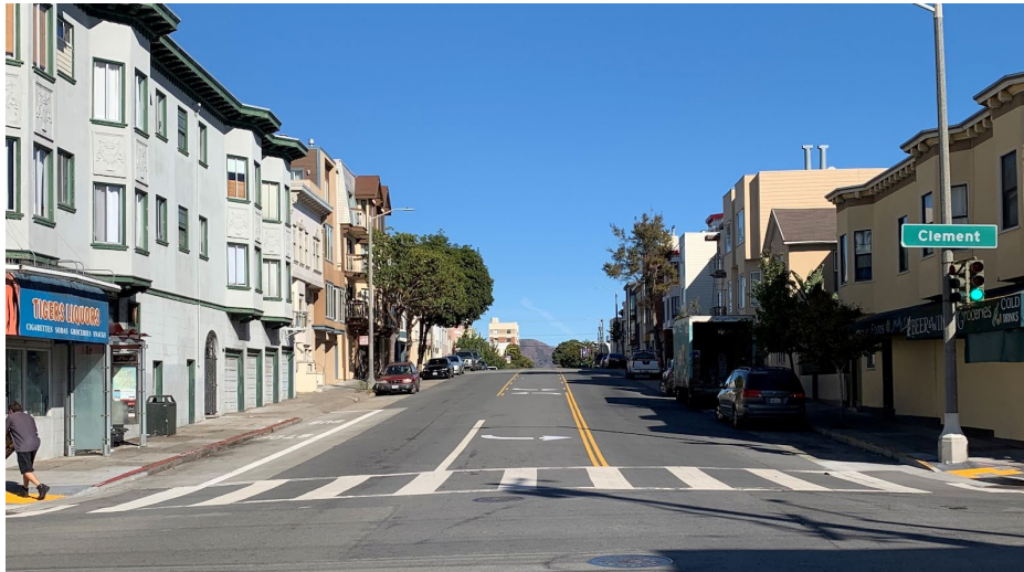
Figure Y. A road diet converts a four-lane street to a three-lane street with a center turn lane.
