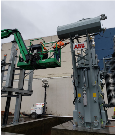
BBI electricians running bus conduits at the transformer and bending the conduits to size for installation at PS-5.
