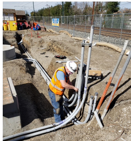
BBI electrician installing PVC conduit for anchoring for concrete pour at PS-5.
