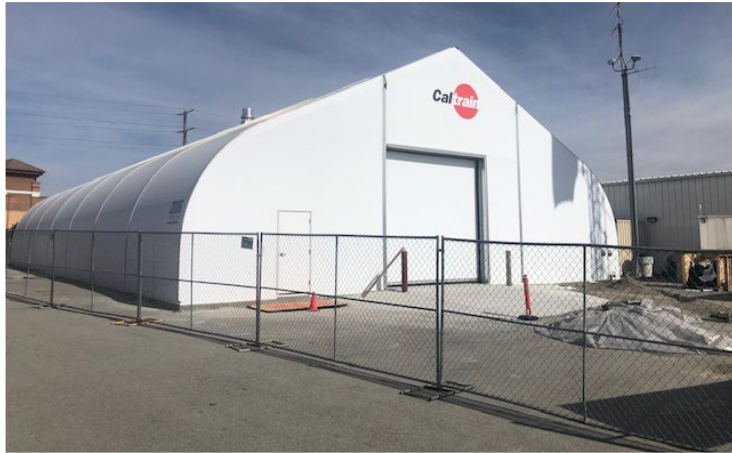
Parts Storage Warehouse
