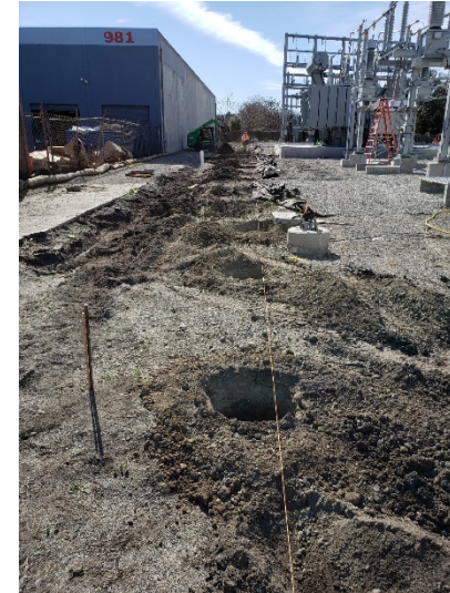
Excavating for site fence foundations at TPS-2.
