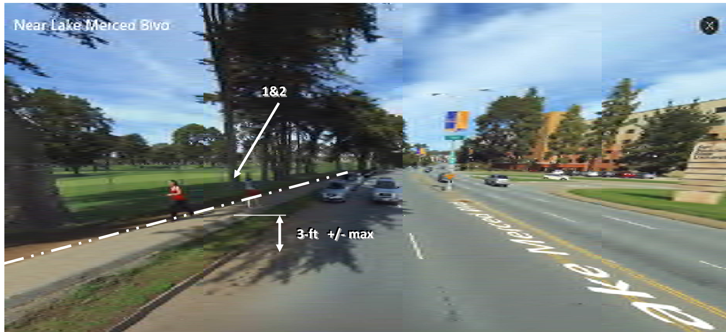
Figure D3 – Lake Merced Blvd at center of raised sidewalk profile (south of Font Blvd)
