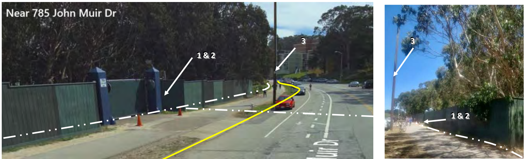
Figure G5 - John Muir Drive, Fence at SF Police Range Site (Entrance looking south and looking north)
