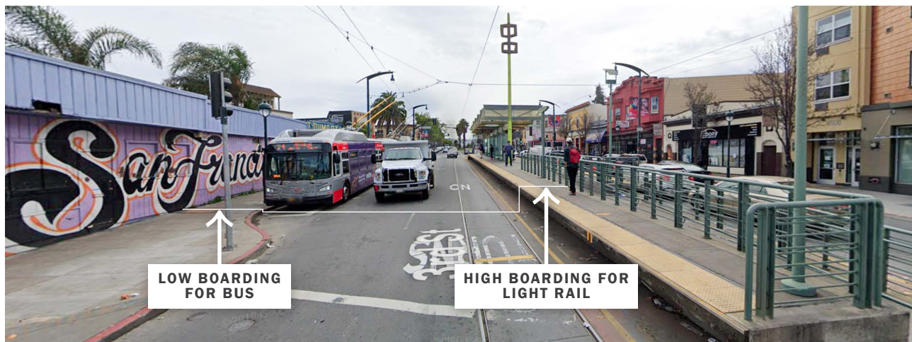
Figure 4-11. T Third and 24 Divisadero Stops at Third and Oakdale
