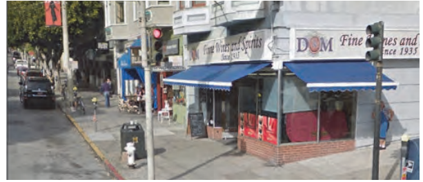
Low profile traffic signals (on existing poles)
