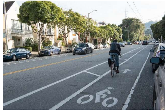
Figure 9 Example of a Buffered Bike Lane
