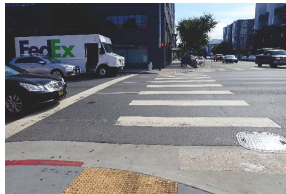
Figure 8 Example of Advance Limit Lines and Continental Crosswalks
