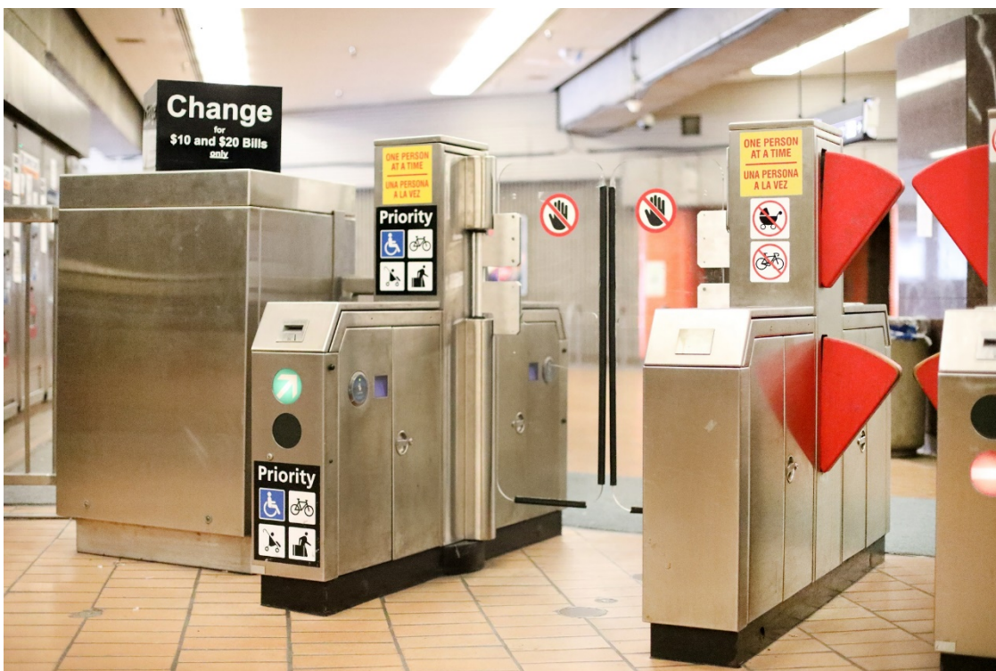
New AFG Installed at BART's Richmond Station
