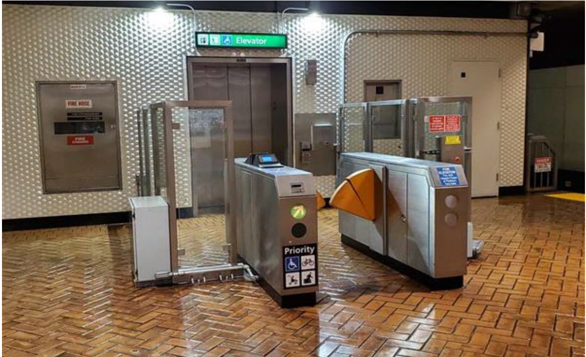
Current AFG located at Montgomery Station, ID M20, Elevator Platform
