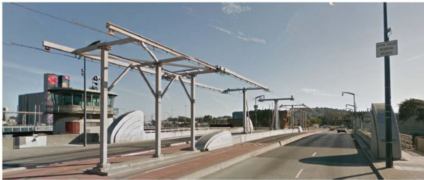
Figure No. 1 – General Overview looking to the South
