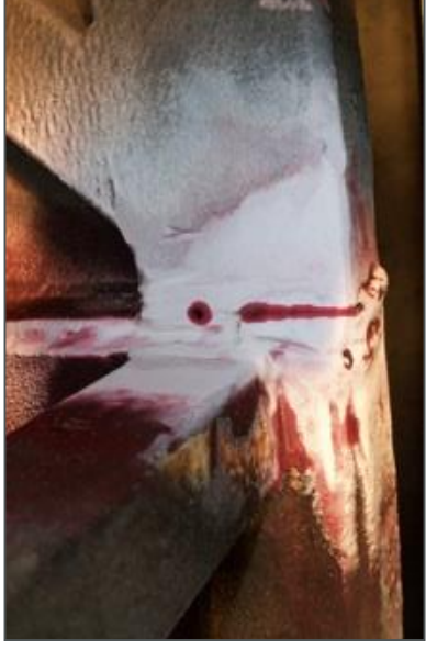
Repaired structural wear
