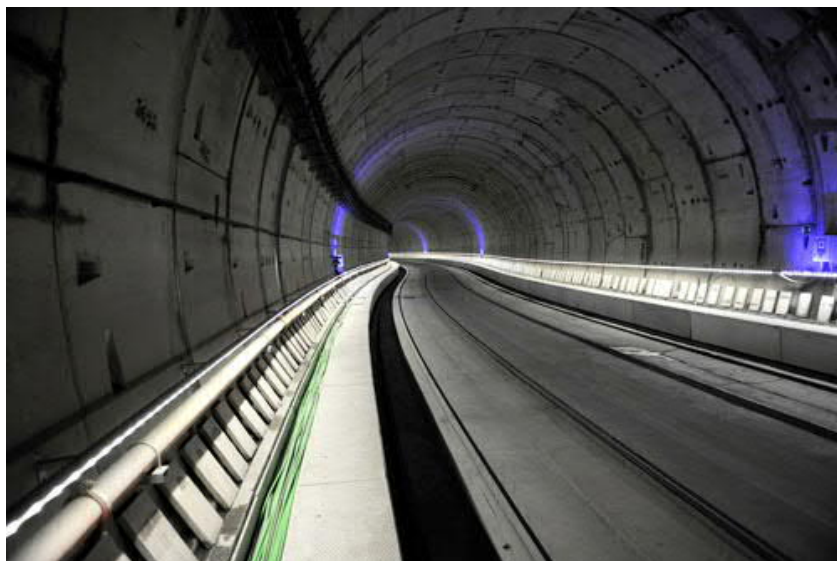
Figure 5: Inside the Atocha Chamartin Tunnel
