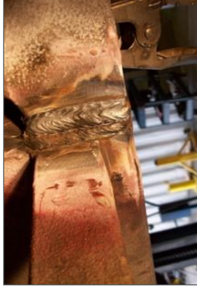
Repaired structural wear
