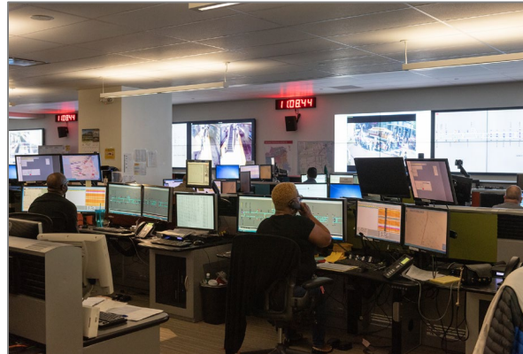
New Transportation Management Center (TMC) and Radio System
