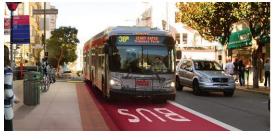
Geary 38 – Ph 1 BRT to break ground in Feb 2019
