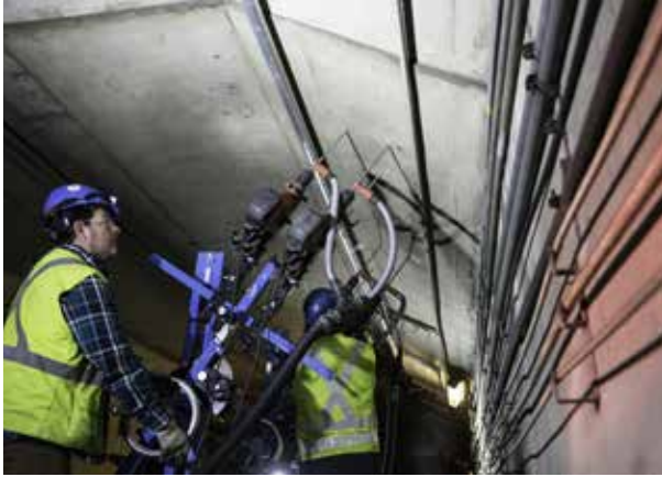
Crews installing brackets to carry communications cables in Twin Peaks Tunnel.
