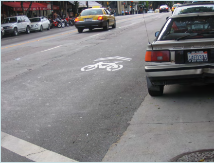
FIGURE 4-22 “SHARROW” MARKINGS DELINEATE AND PROTECT SPACE FOR CYCLISTS ON A SHARED ROADWAY.
