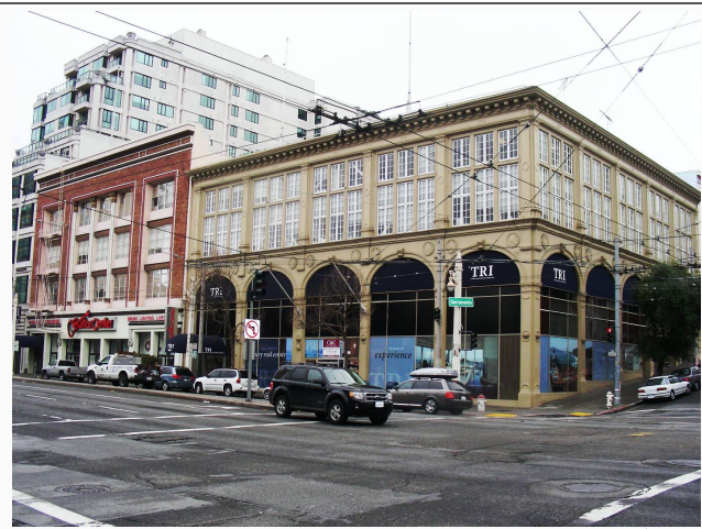
H-6: Paige Motor Car Co, 1699 Van Ness Avenue, Facing Southwest from Van Ness Avenue
