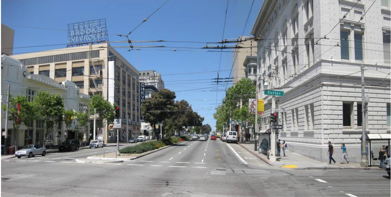
Existing Conditions at Van Ness Avenue and Sutter Street Intersection
