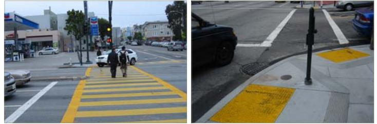
Key to the *Transportation Plan's* recommendations is traffic controllers that support pedestrian countdown signals, better signal coordination, and transit signal priority, necessitating replacement of the current, outdated equipment. In addition to new traffic signals, the project will provide pedestrian countdown signals, Americans-with-Disabilities-Act-compliant curb ramps, and re-striped crosswalks.
