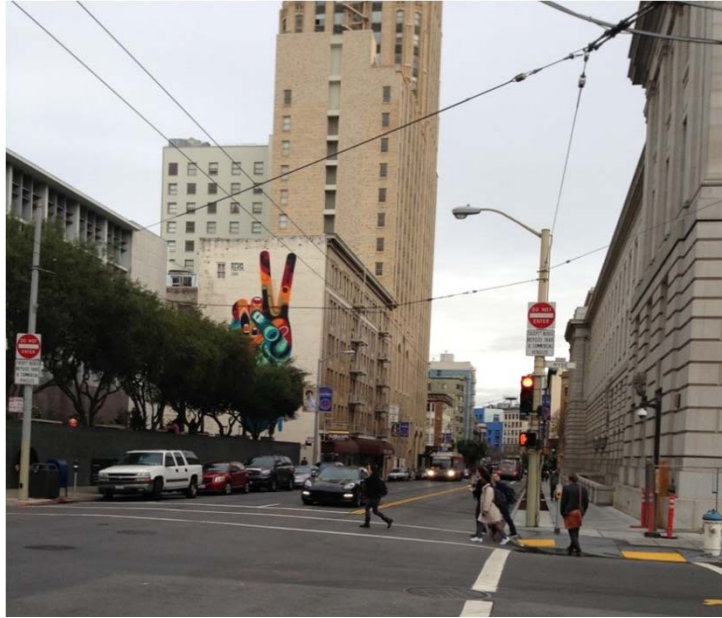
100 Block of McAllister Street Looking Eastward, Project Area on the Left
