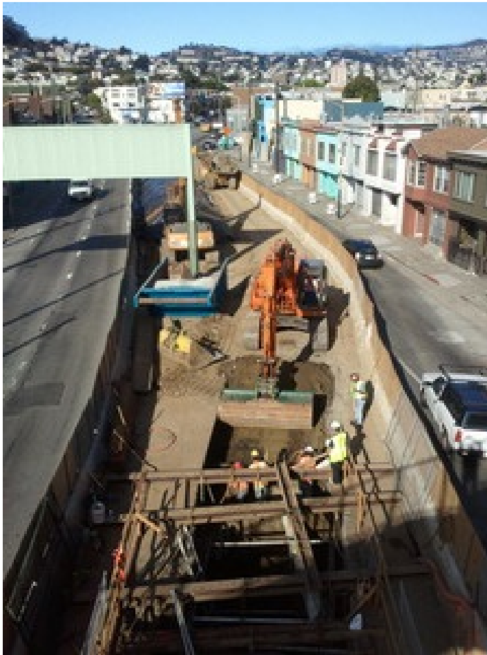
Cesar Chavez construction
