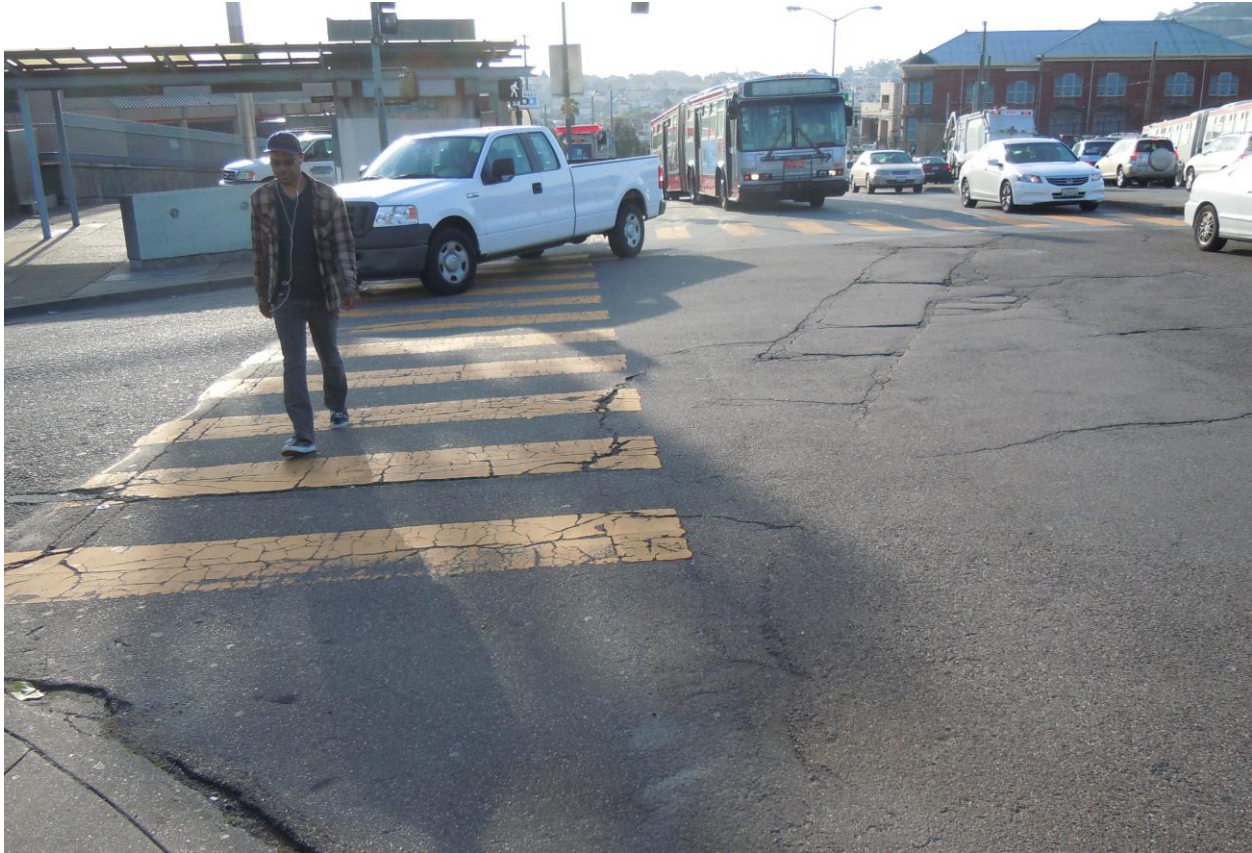
Figure 2: Intersection at Geneva Avenue and I-280 NB On-Ramp
