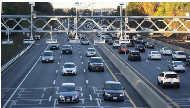
1 All-Lane Highway Tolling
