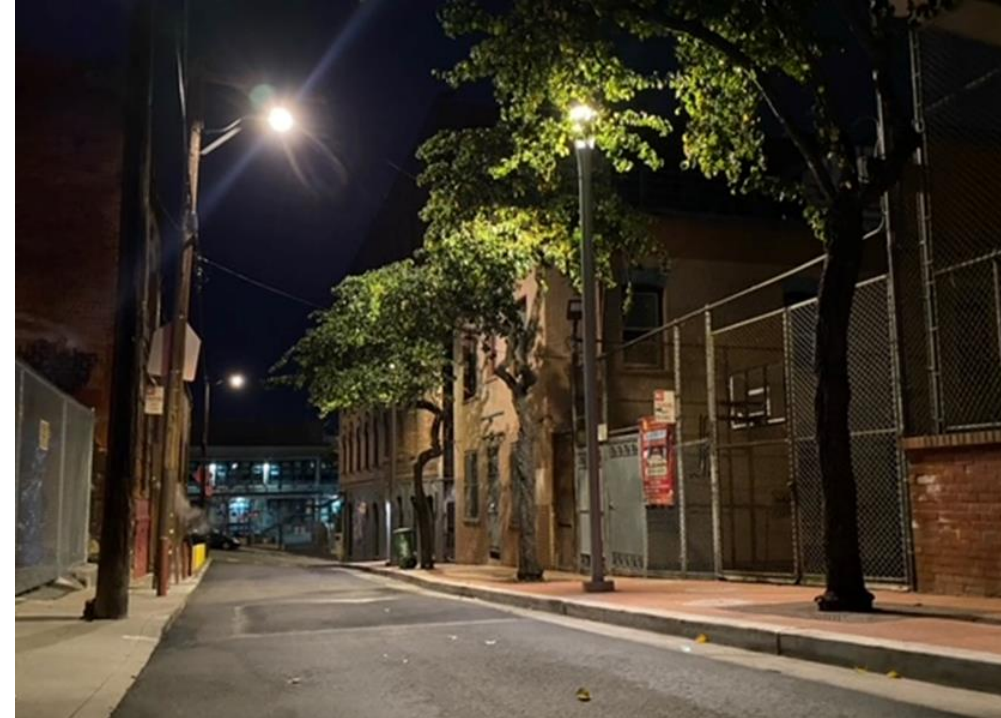
SFPW's recently completed Joice Alley Lighting Improvements, funded by Prop AA
