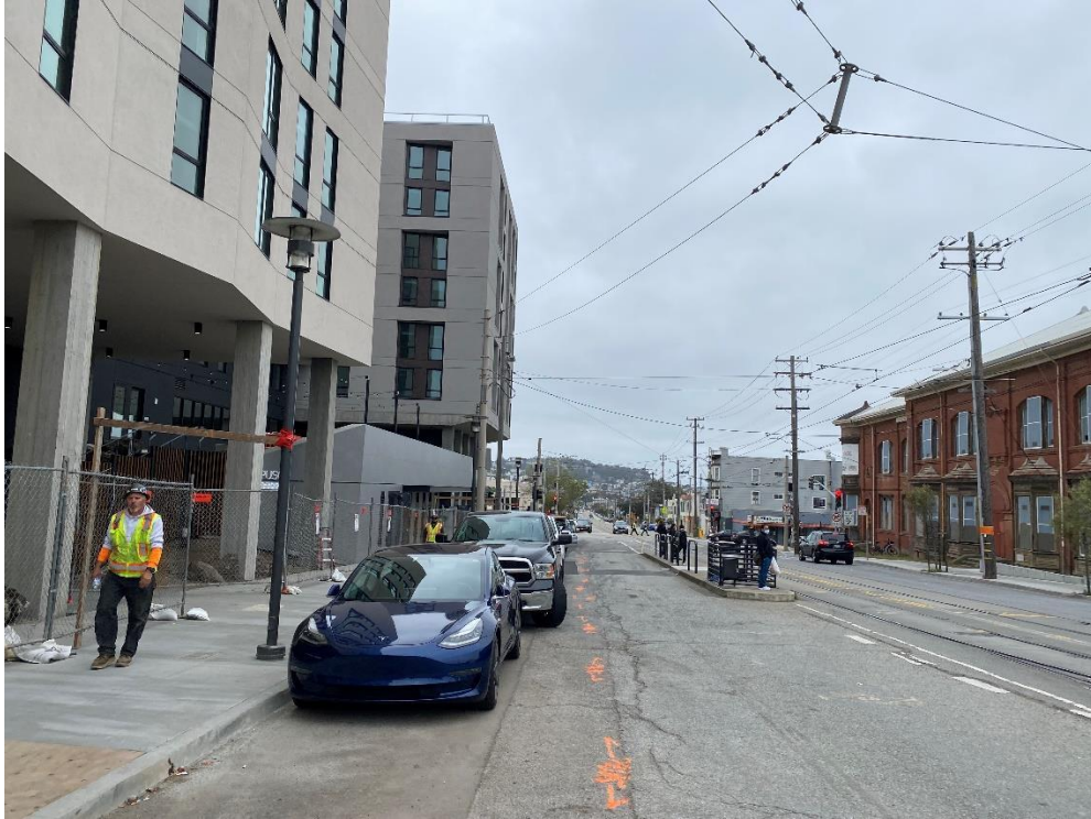
Figure 3. Existing M ocean View first inbound boarding island on San Jose Avenue, facing Geneva Avenue
