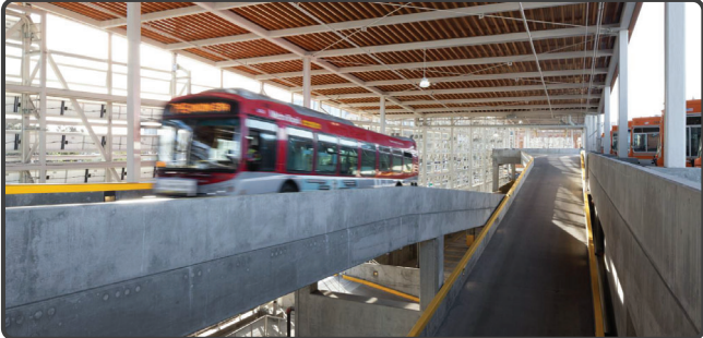
Circulation Ramps: Main circulation area that allows vehicles to move up and down between floors.
