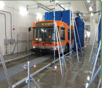
Bus Washer/Water Reclamation: Dedicated area for automatic washing of sides, top, front, and under carriage of the trolleys, motor coaches and BEB's.
