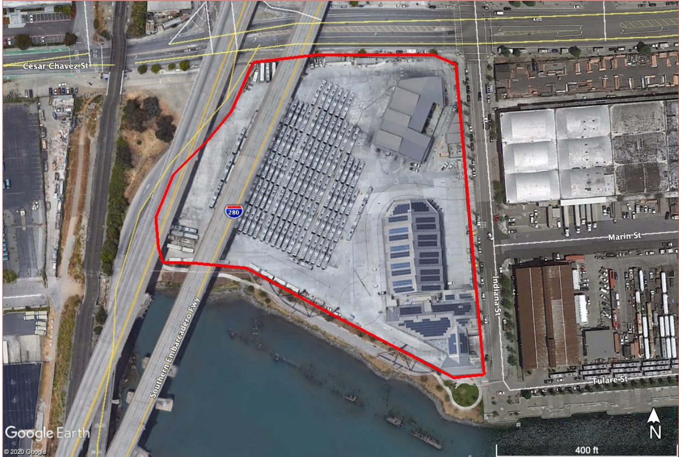
Figure 5-1. Islais Creek Yard – Existing Conditions (Aerial)
