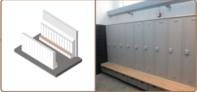
Maintenance Staff Lockers: Locker area for male and female Bus Maintenance employees.
