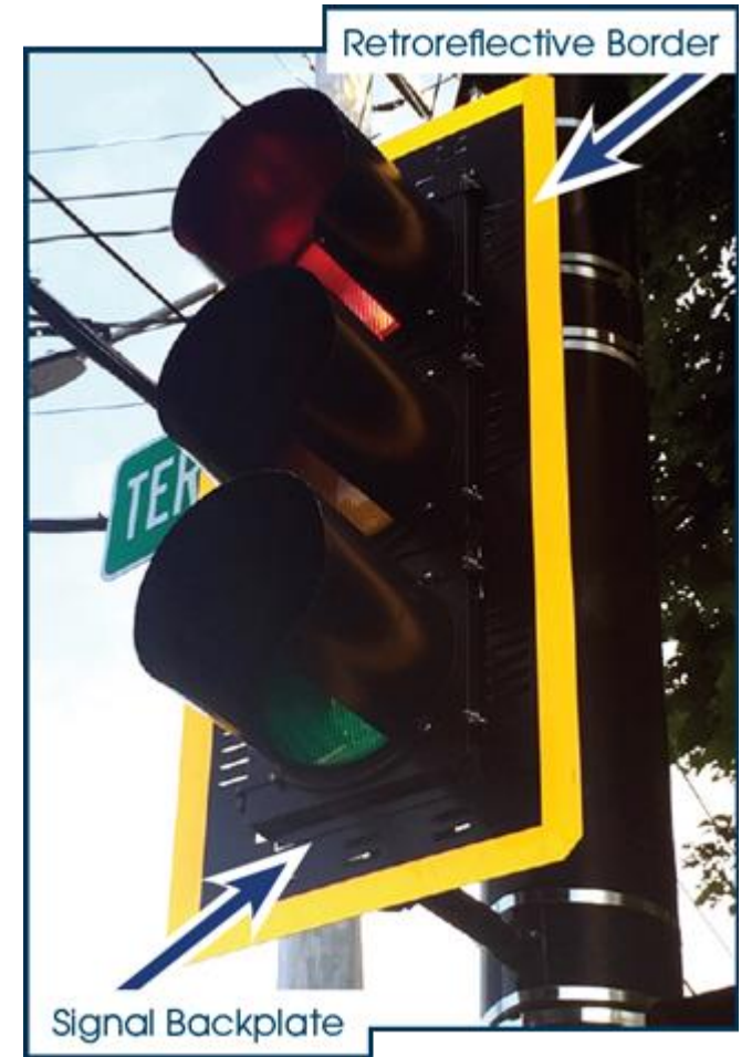
Signal backplate framed with a retroreflective border. Source: FHWA
