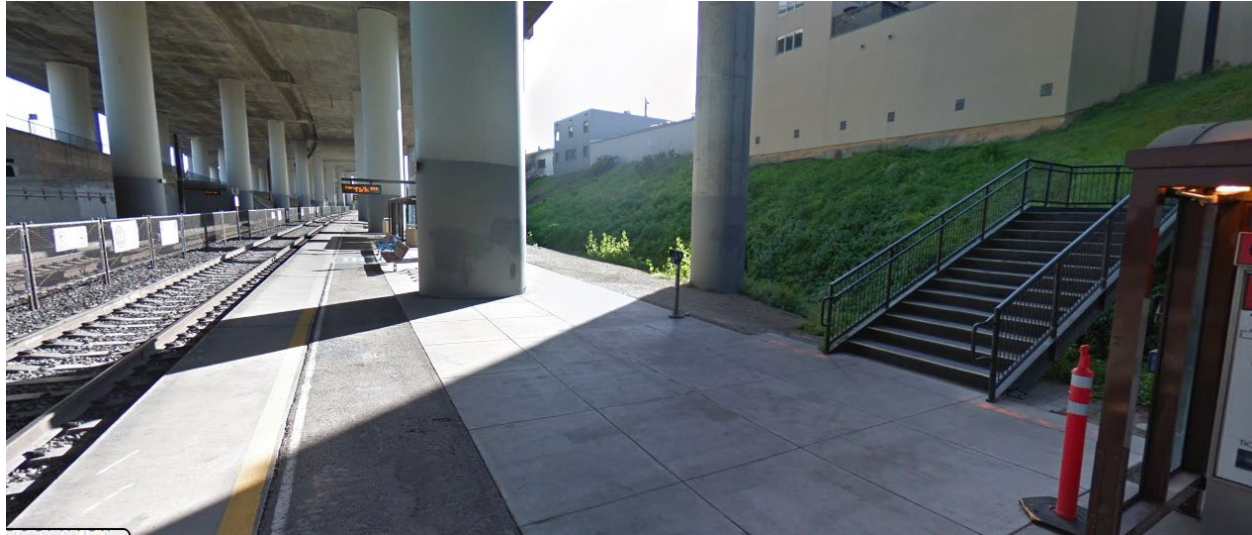
Figure 10 Southbound Platform Looking Southward from TVM
