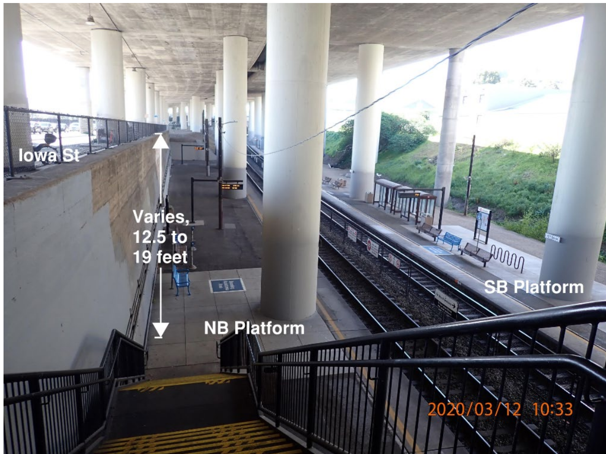
Figure 2 Northbound Platform, Facing South from the Top of the Staircase
