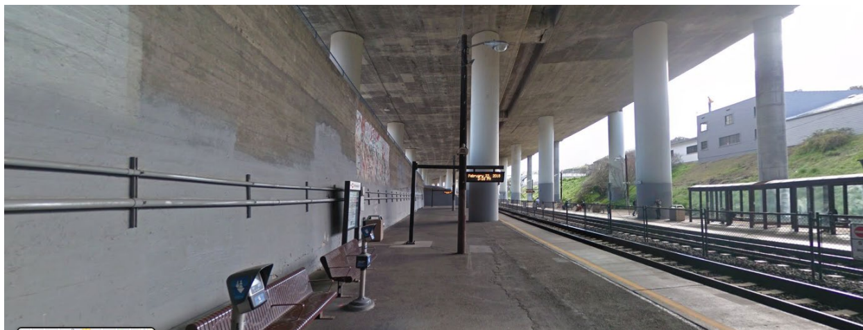
Figure 3 Northbound Platform Retaining Wall
