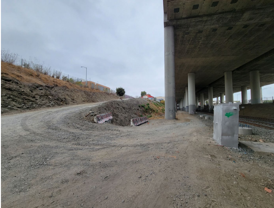
Figure 8 Southbound Platform Gravel Access Road
