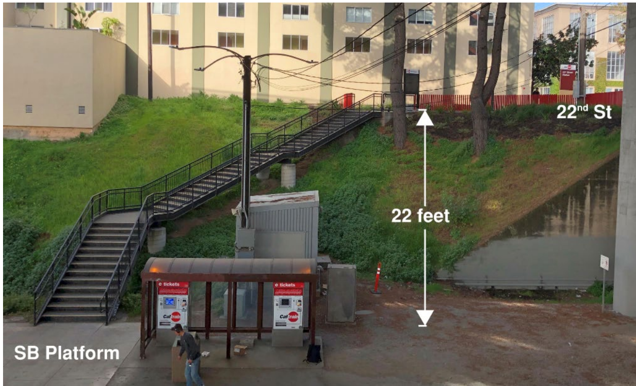
Figure 9 Southbound Platform Staircase
