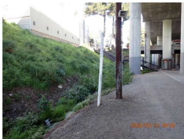
Figure 12 Southbound Platform Drainage Ditch
