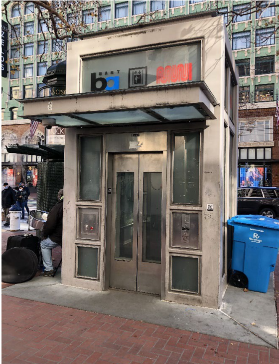
Figure 6. Street elevator at Powell St. Station, December 2021.
