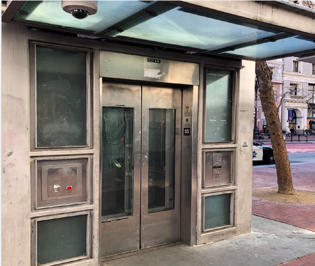
Elevator Modernization Project, Phase 1.3 Powell Street and Civic Center/UN Plaza Stations
