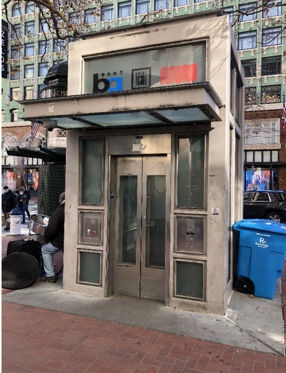
Figure 6. Street elevator at Powell St. Station, December 2021.
