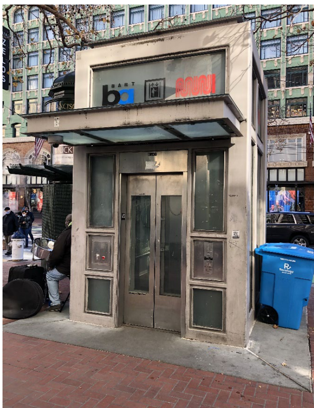
Figure 5. Street elevator at Powell St. Station, December 2021.
